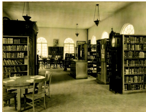
Shows the original interior of the Carnegie Building. The main beam is under this 15 foot span.
